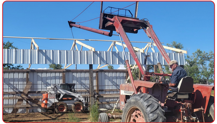
Repairing Storm Damage with a New Roof
